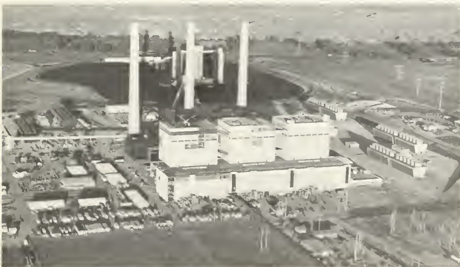
This 1.5-million kilowatt plant near Wheatland, Wyo., is owned by six co-op and municipal wholesale power organizations. Its lines ultimately serve about 2 million people throughout an eight-State region.
